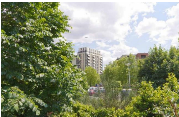
LEFT: Lend Lease image of Empire House Tower from behind the bushes
